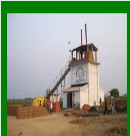
Vertical Shaft Brick Kiln (VSBK)
